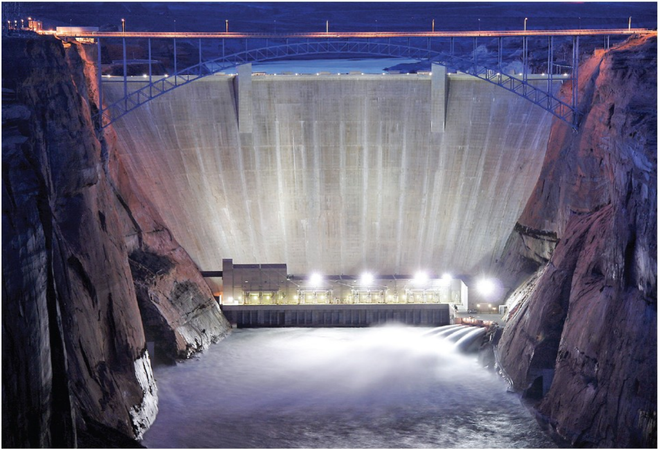
Figure 11.8: Glen Canyon Dam in March 2008 during a controlled flood with increased release of water. Source: Melis et al. 2010
