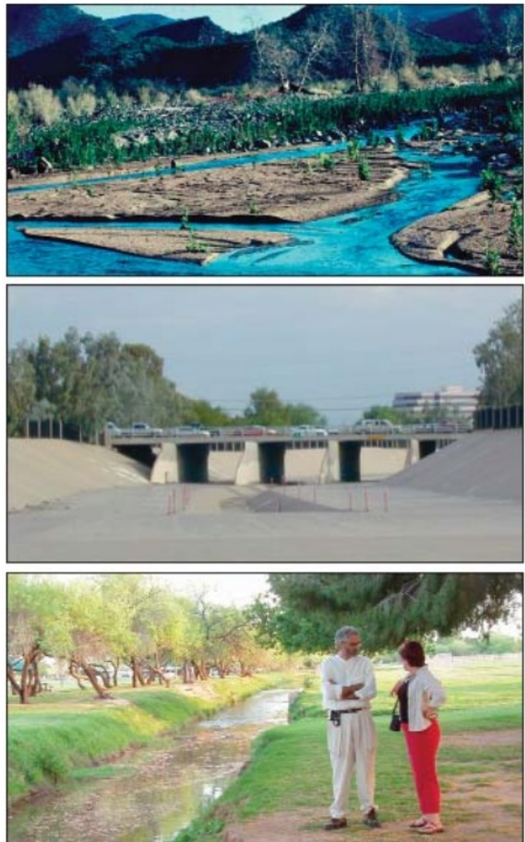
Figure 9.2: Application of ecological engineering principles. In the desert southwest, natural stream flow (top) varies but may increase substantially after large summer rainfall events. A common past solution has been to convert stream channels to concrete culverts (middle). This reduces economic loss from flooding but provides few other ecological, social, or economic benefits. An alternative to concrete is an ecological engineering solution, such as Indian Bend Wash in Scottsdale, AZ (bottom), in which vegetated pathways and wetlands minimize flood damage, improve water quality, enhance surrounding land values, and create a park-like environment for recreational activities. Source: Palmer et al. 2004
